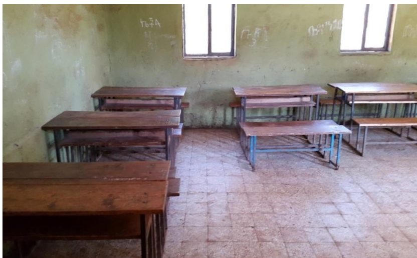
Figure 4.8. One of the elementary school classroom blocks (top) and a classroom (bottom) renovated in 2011 (photos taken in 2015).
