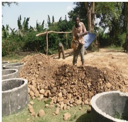
Digging a well.
