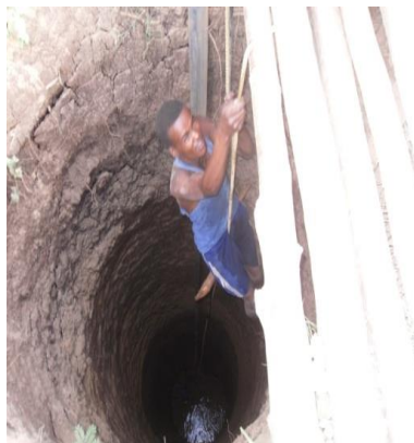
Discovering a good water level.
