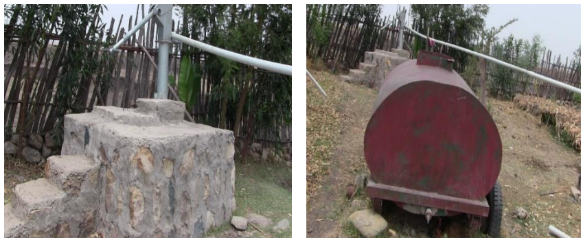
Figure 3.4. Hand-dug well on raised stone platform (left), water collection tanker and supply line (right) in Kersole.
