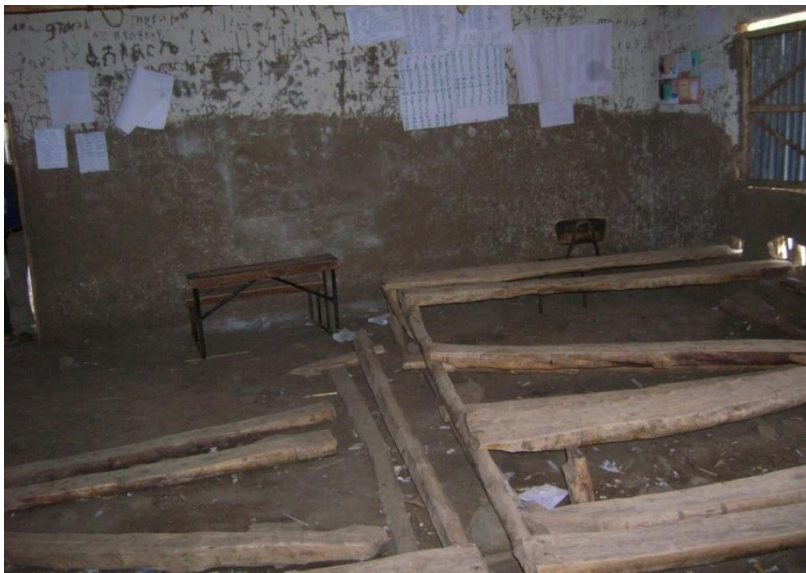
Figure 4.7. Two elementary school classrooms before renovation.
