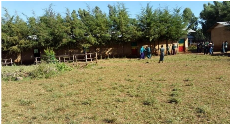
Figure 4.9. Surroundings of some of the renovated buildings.
