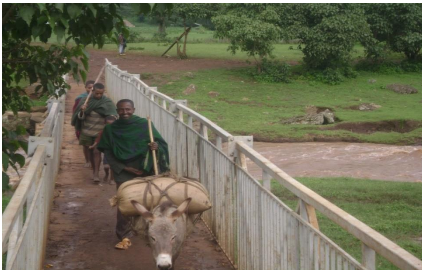
Figure 4.4. Daily traffic on the bridge.
