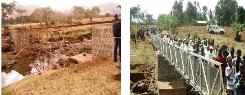
Figure 4.3. The bridge under construction and during the opening ceremony in May 2009.
